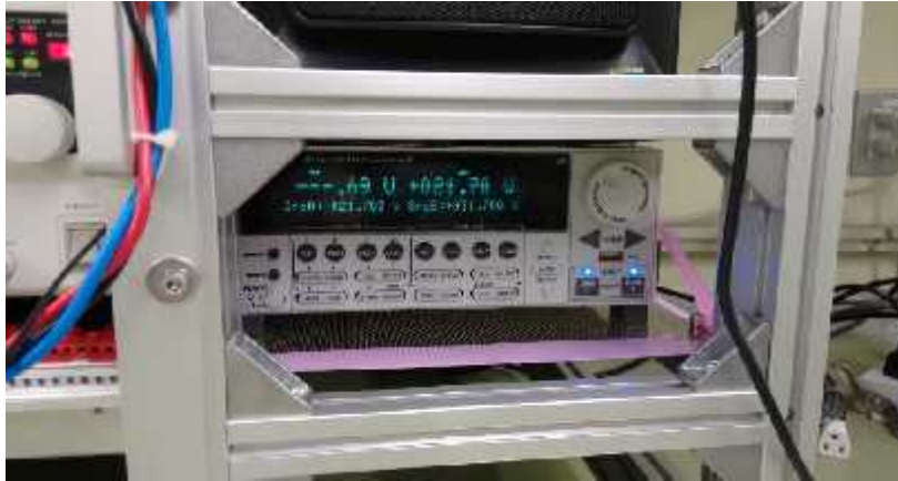
High voltage power supply
