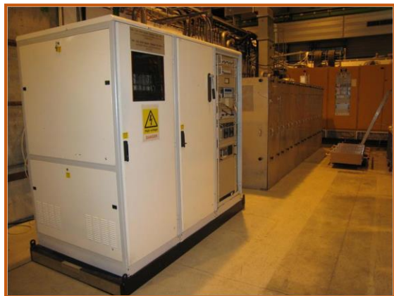
100kV solid state modulator designed, developed and commissioned by RRCAT, Indore, for LINAC 4 cavity tests.
