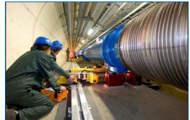
Installation of dipoles on Indian jacks
