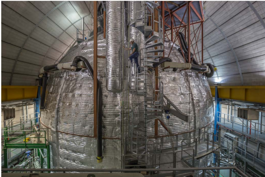
Borexino Water Tank after the completion of the thermal insulation layer
