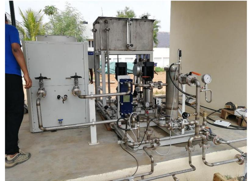
**Low conductivity water cooling system for magnet & power supply**
