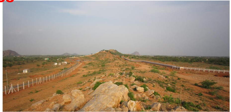
Inter-Institutional Centre for High Energy Physics (IICHEP), Madurai
