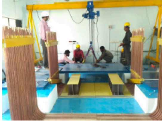
Magnet assembly in progress
