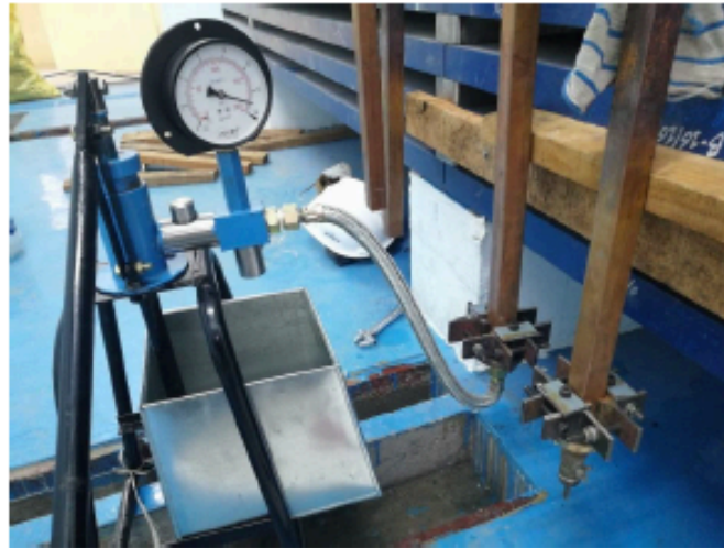
Coil hydrostatic pressure test
