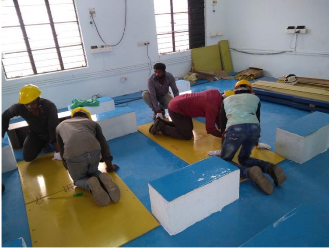
Pillars for magnet, G10 boards for Cu coils
