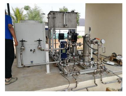
Low conductivity water cooling system for magnet & power supply
