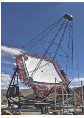
Fig.5 A photograph of the telescope with 225 mirror panels, depicting the present status of the MACE telescope.
