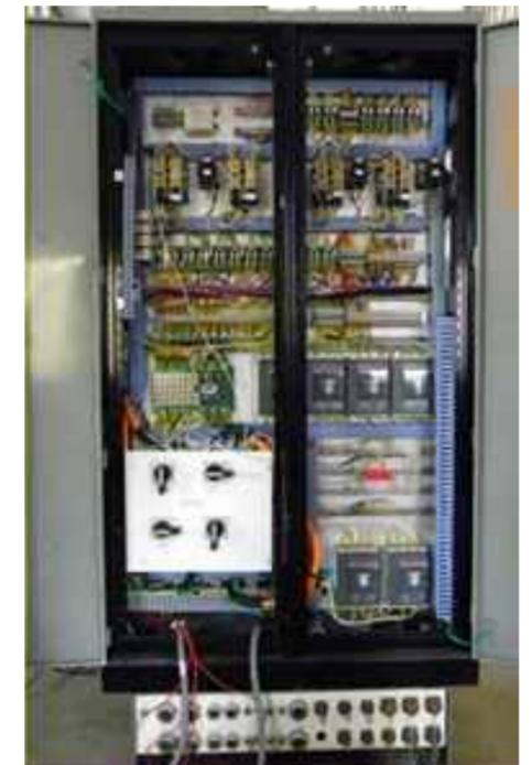
Fig.6 A photograph of the drive control unit of the telescope.
