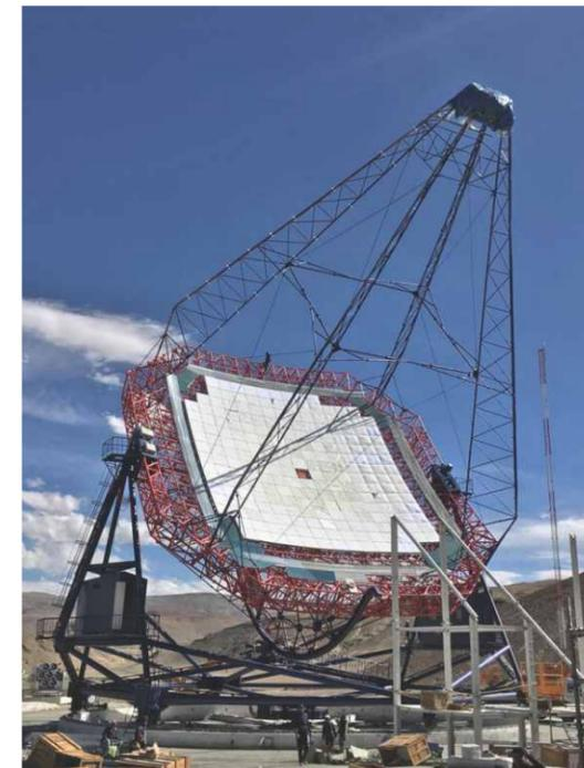
Fig.5 A photograph of the telescope with 225 mirror panels, depicting the present status of the MACE telescope.
